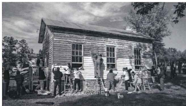
Community renovating Ashburn school
